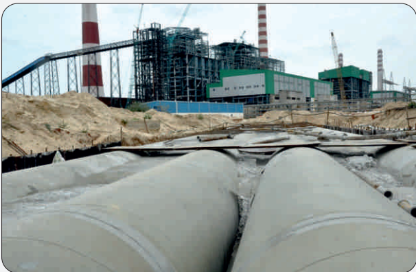
Coated pipeline under installation
