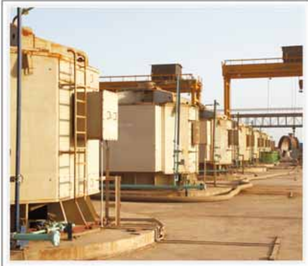
Concrete volute pump ready to start at Coastal Gujarat Power Limited, Mundra
