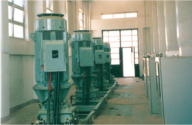
Vertical Turbine Pumps installed at Wadi Sheeh
