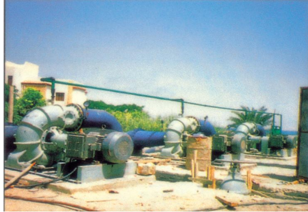
Mixed Flow Pumps for sewage application at Faiyad, Egypt
