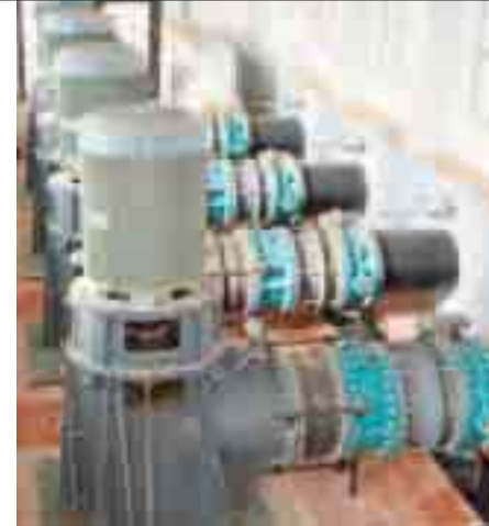
Diar Abu Hennes - Intake Pumping Station, four BHM 55 Pumps with 240 kW Motor (Capacity - 1.65 m 3 /sec @ static head of 8.47 m)
