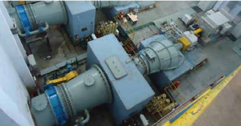
Darna HEP, Maharashtra, India Type of turbine: Horizontal ‘S’ Type tubular Kaplan Turbine Project capacity: 2 x 2450 kW Application: Electricity generation from dam based hydro power station
