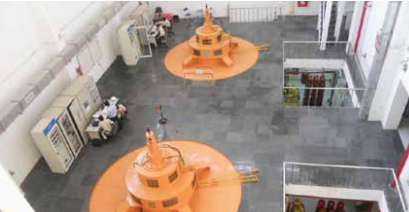
Ankhe Kanak, Vietnam Type of turbine: Vertical Kaplan Turbine Project capacity: 2 x 6500 kW Application: Electricity generation from run-off the river hydro power station
