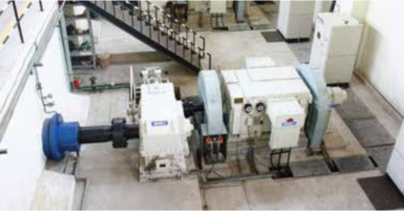
RanniPerunad, Kerala, India Type of turbine: Horizontal ‘S’ Type tubular Kaplan Turbine Project Capacity: 2 x 2000 kW Application: Electricity generation from run-off river type hydro power station
