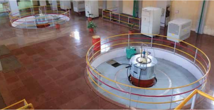
Konal HEP, Maharashtra, India Type of turbine: Vertical Kaplan Turbine Project Capacity: 2 x 5500 kW Application: Electricity generation from dam based hydro power station
