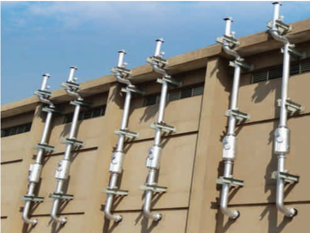
External surface coating done on exhaust pipes to withstand thermal cyclic shocks and prevent corrosion for a LNG regassification Terminal
