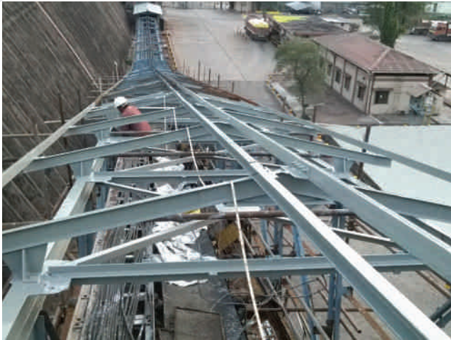
Structural coating for a Coastal Fertilizer Plant
