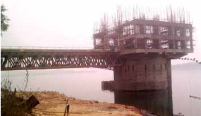
Intake well for Raw Water at Tilaya Dam
