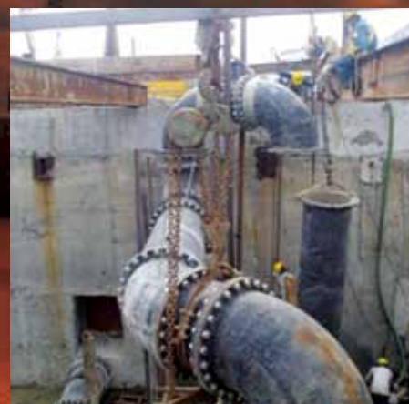
Installation of Ductile Iron (DI) pipes with help of chain pulley blocks and makeshift arrangements of supports
