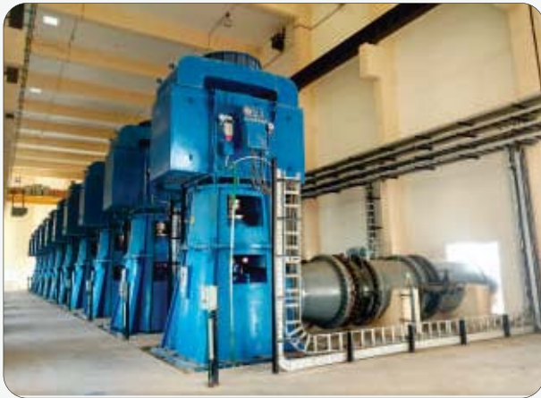
Kirloskar Vertical Turbine pumps installed at Sauni Yojana Project, Botad, Gujarat
