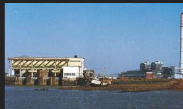
(India's first Concrete Volute Pumps)
