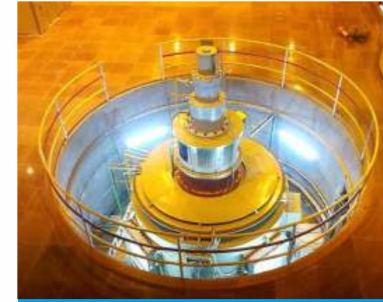
ERECTION OF VERTICAL GENERATOR
