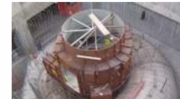
ERECTION OF CASING & PIT LINER
