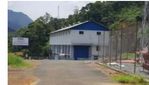
BARAPOLE HEP, 3 X 5 MW, KERALA
