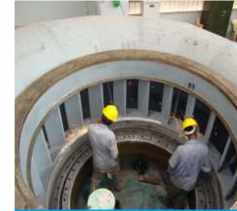
ERECTION OF STAY RING
