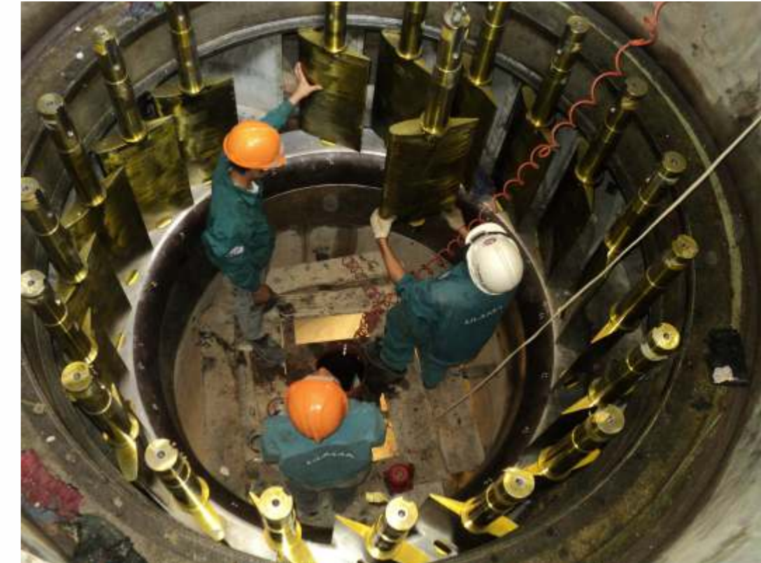
GUIDE VANE ASSEMBLY AT SITE
