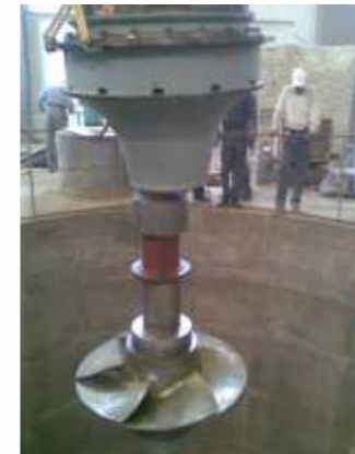
ERECTION OF VERTICAL KAPLAN RUNNER
