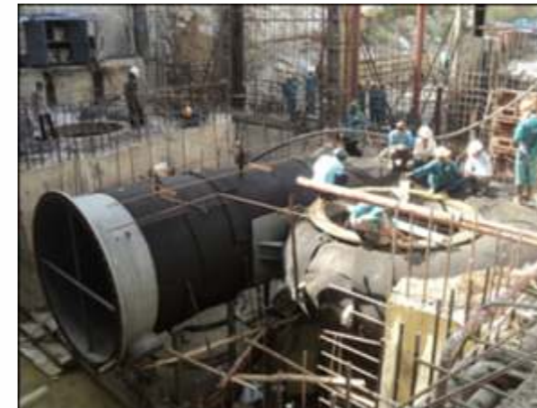
ERECTION OF SPIRAL CASING
