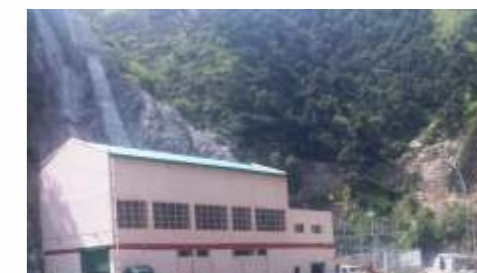
PANWI HEP, 2 X 2 MW, HIMACHAL PRADESH
