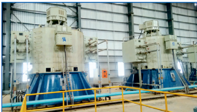
Vertical Turbine pumps installed at Pattiseema project
