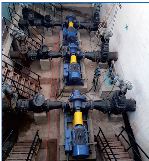
LLC Pumps installed at Delhi Jal Board
