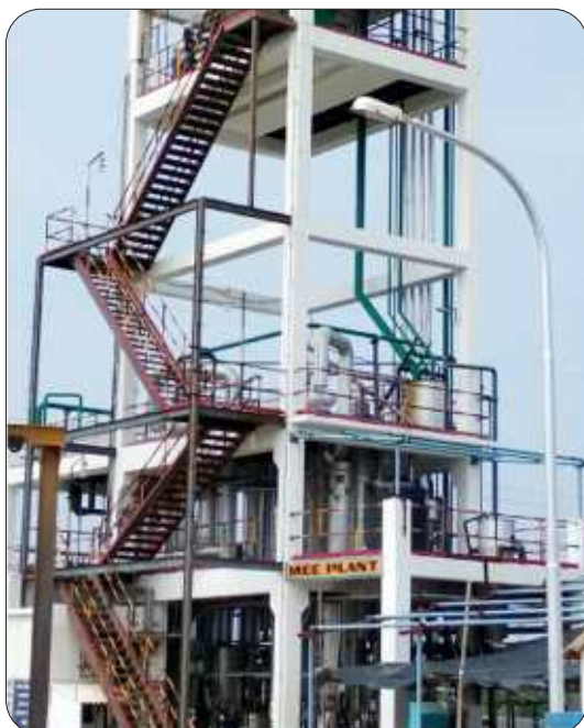
Structures coated with Plasmert ZF and Plasmert ZE epoxy glass flake coating system for providing long term corrosion protection
