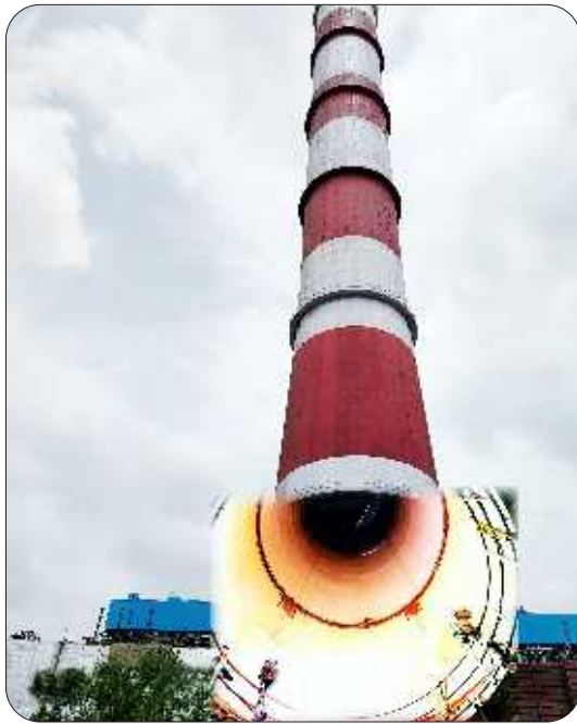
Chimney Flues internally coated with Corothane XT – a high temperature resistance coating
