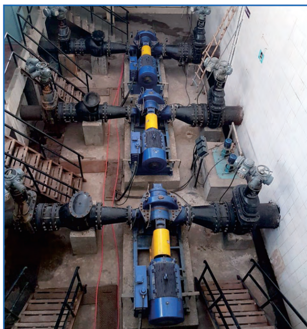
LLC Pumps installed at Delhi Jal Board
