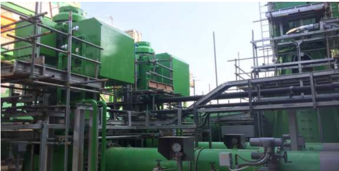
KBL CW Pumps installed onsite at Mae Moh Power Plant, Thailand
