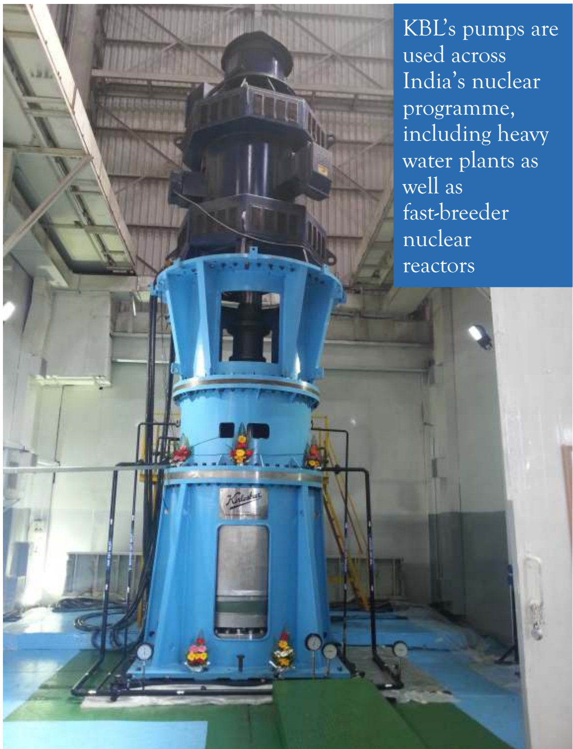
(Actual On-site Image) Kirloskar Primary Sodium Pump installed at BHAVINI'S Atomic Power Station at Kalpakkam, Tamil Nadu
