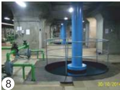
8 Assembly of Transmission shaft with Pump Coupling Hub
