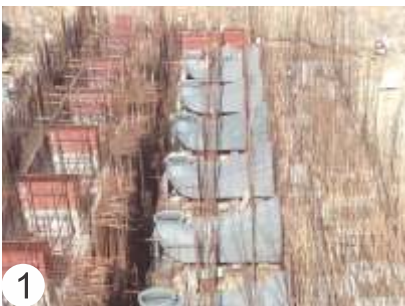
1 Placement of Suction Draft Tube, anchoring and concreting
