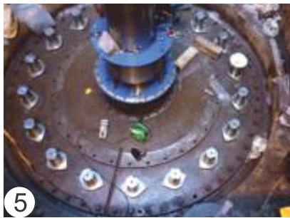
5 Placement of Head Cover Sub-Assembly on Spiral Casing
