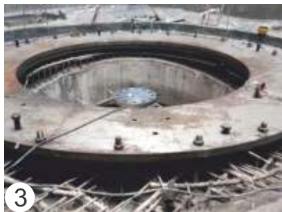
3 Placement of Motor Base Plate on motor floor level for motor or gear box or motor stool and grout it.
