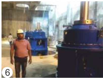
6 Placement of Journal Bearing Unit and thrust Bearing Unit on Head Cover
