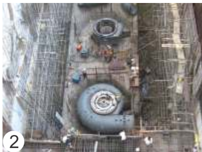
2 Placement of Spiral Casing, Suction Cone and Bottom Cover. Anchoring and Concreting
