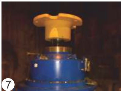
7 Assembly of Coupling Hub with Pump Shaft and Motor Shaft
