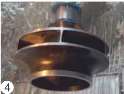
4 Placement of Rotating Unit Sub-Assembly in spiral casing
