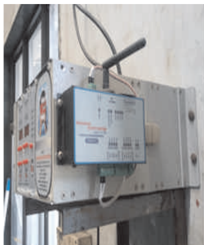
Use of IOT in operations (Ammonia Gas Detection System with SMS Alert)
