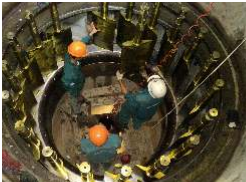
Guide Vane Assembly at Site
