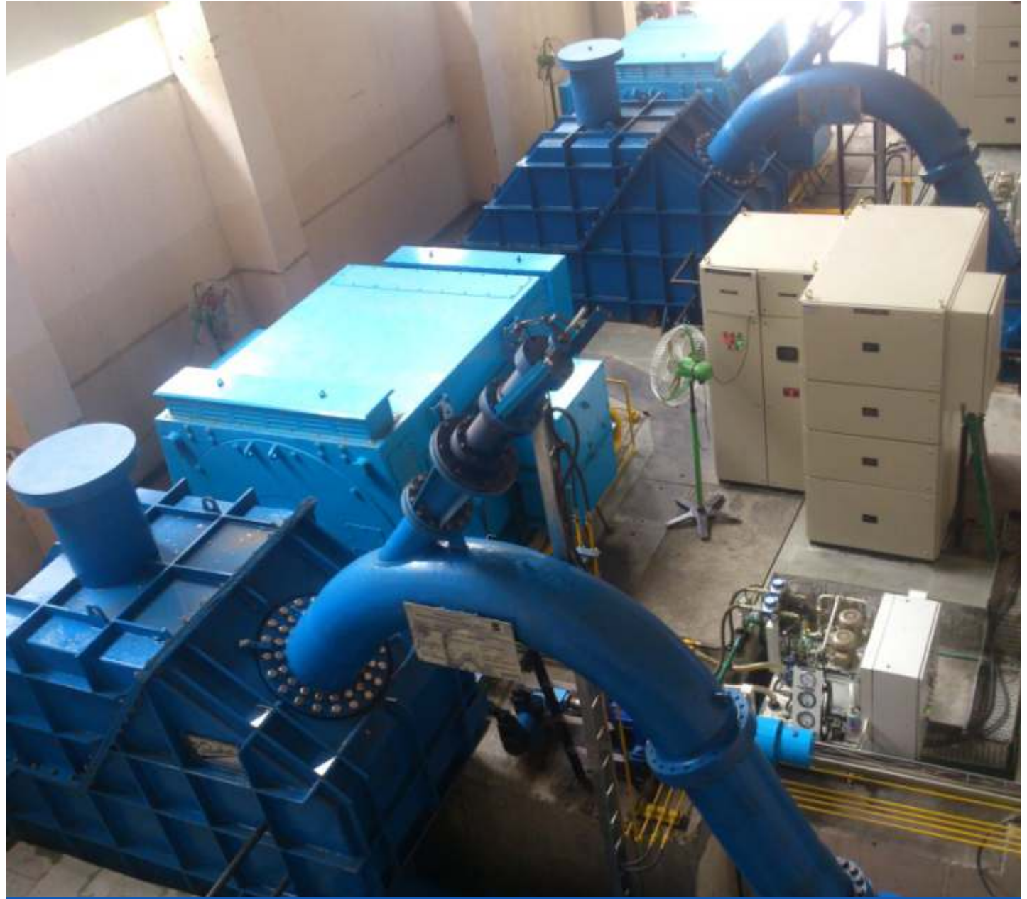
Panwi HEP 2 X 2 MW, Twin Jet Pelton Turbine
