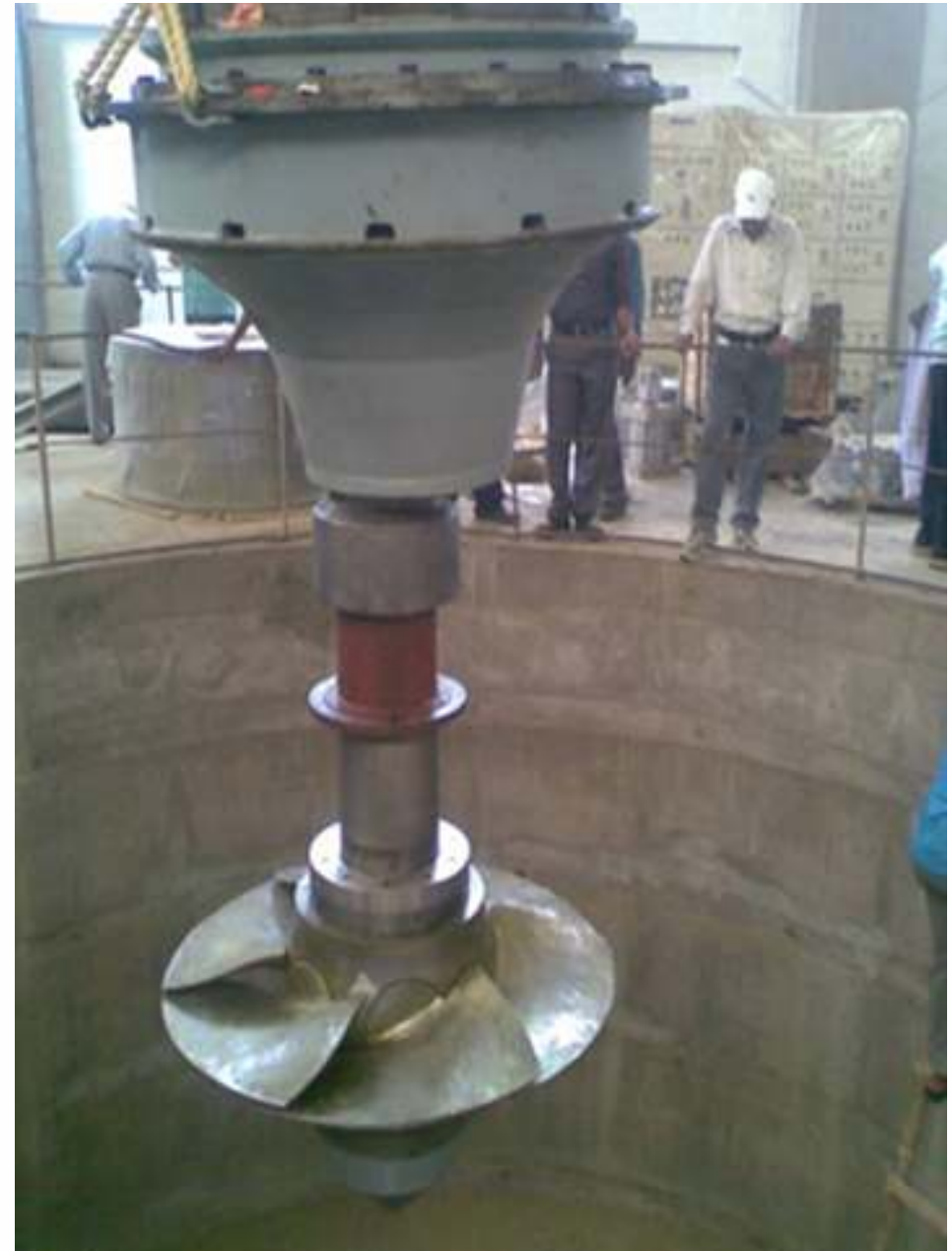
Erection of Vertical Kaplan Runner
