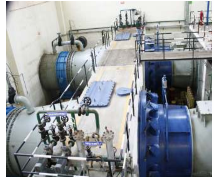
Ranni Perunad HEP, 2 X 2 MW, Horizontal 's' Type Tubular Kaplan Turbine
