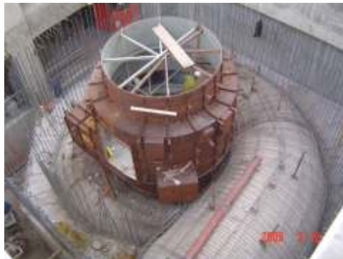
Erection of Casing & Pit Liner
