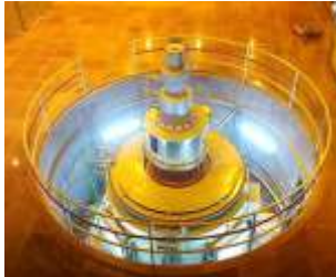
Erection of Vertical Generator
