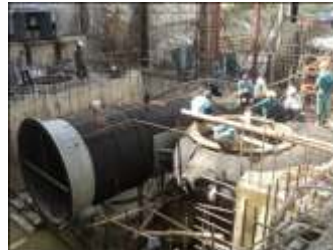
Erection of Spiral Casing
