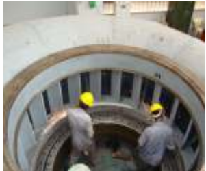
Erection of Stay Ring
