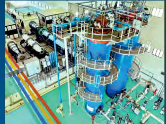
Supply of Multi-stage Multi-outlet (MSMO) – RKB pumps for the world's third-largest hypersonic wind tunnel commissioned by ISRO at Vikram Sarabhai Space Centre, Thiruvananthapuram
