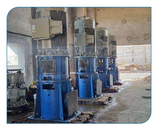
Kirloskar Brothers Limited (KBL) continues to drive progress in rural India by ensuring water accessibility for agricultural communities. As part of the Nizamsagar Project, KBL has successfully installed four Vertical Turbine (VT) pumps for the Irrigation and CAD Department in Telangana. These pumps are a key component of the lift irrigation scheme designed to provide much-needed water supply to Jakora and Chandur.
