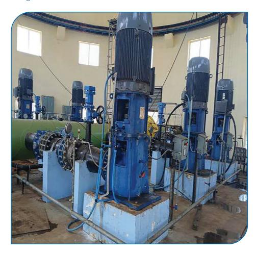
KBL has once again demonstrated its engineering excellence with the successful commissioning of five Vertical Turbine (VT) pumps and three Horizontal Split Case (HSC) pumps for the Payli Water Supply Scheme (WSS) in Jabalpur, Madhya Pradesh.
