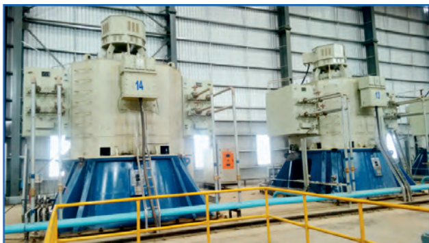
Vertical Turbine pumps installed at Pattiseema project
